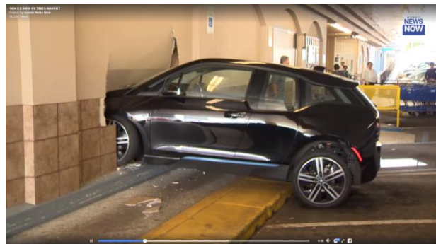
Figure 32. Side view showing damage to the wall behind the parking space. Store entrance is in the background. 47
